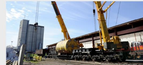
Special and Project transports
