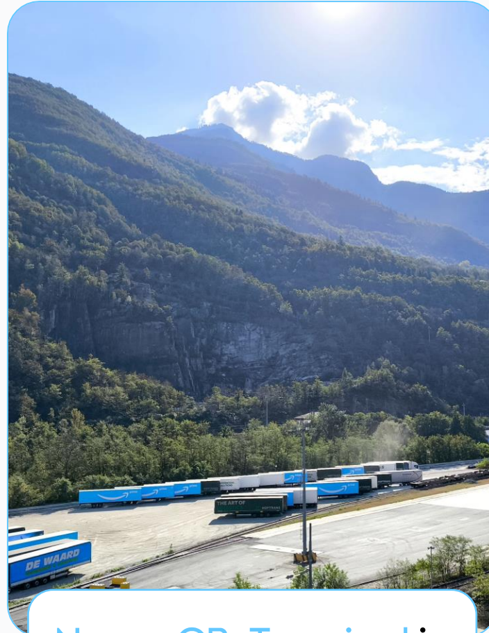
Neues CB-Terminal in Domodossola (IT)
